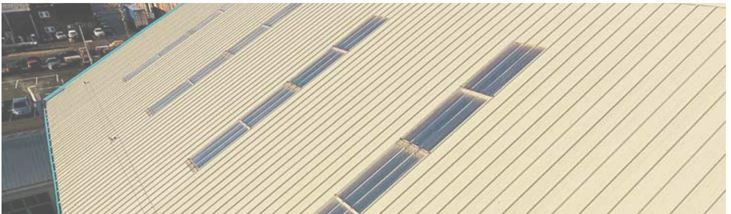
Completed roof and rooflight installation
