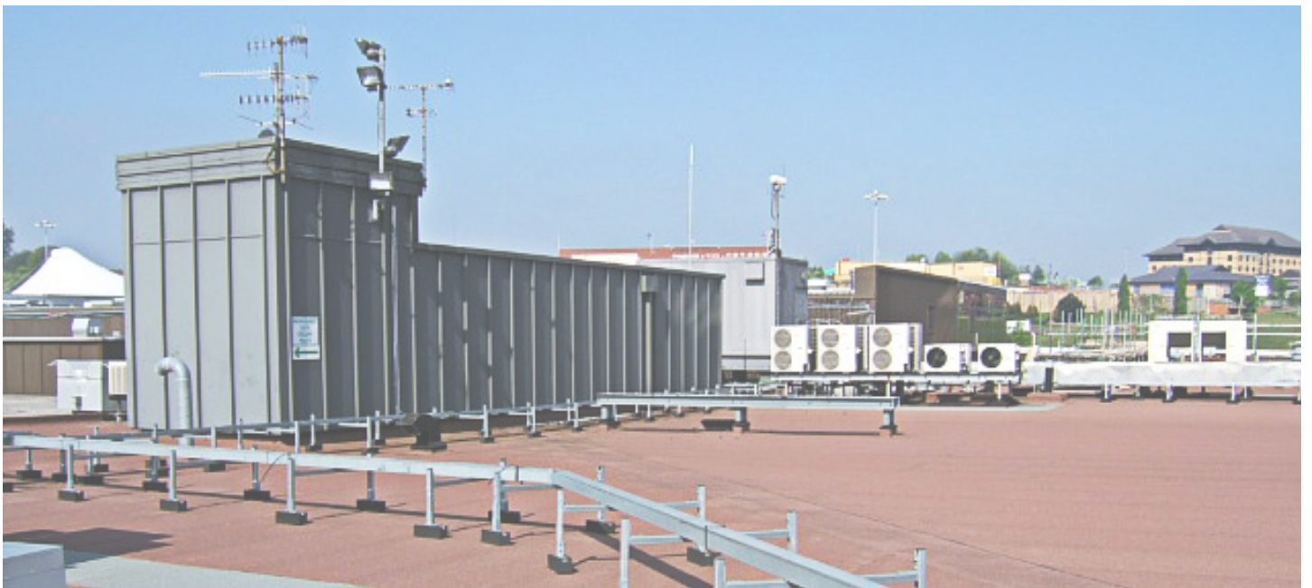
New cable management support structure installed allowing ease of roof maintenance
