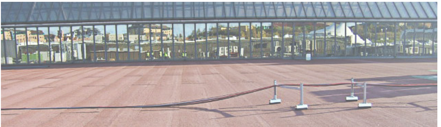
Cable mangement tray being installed
