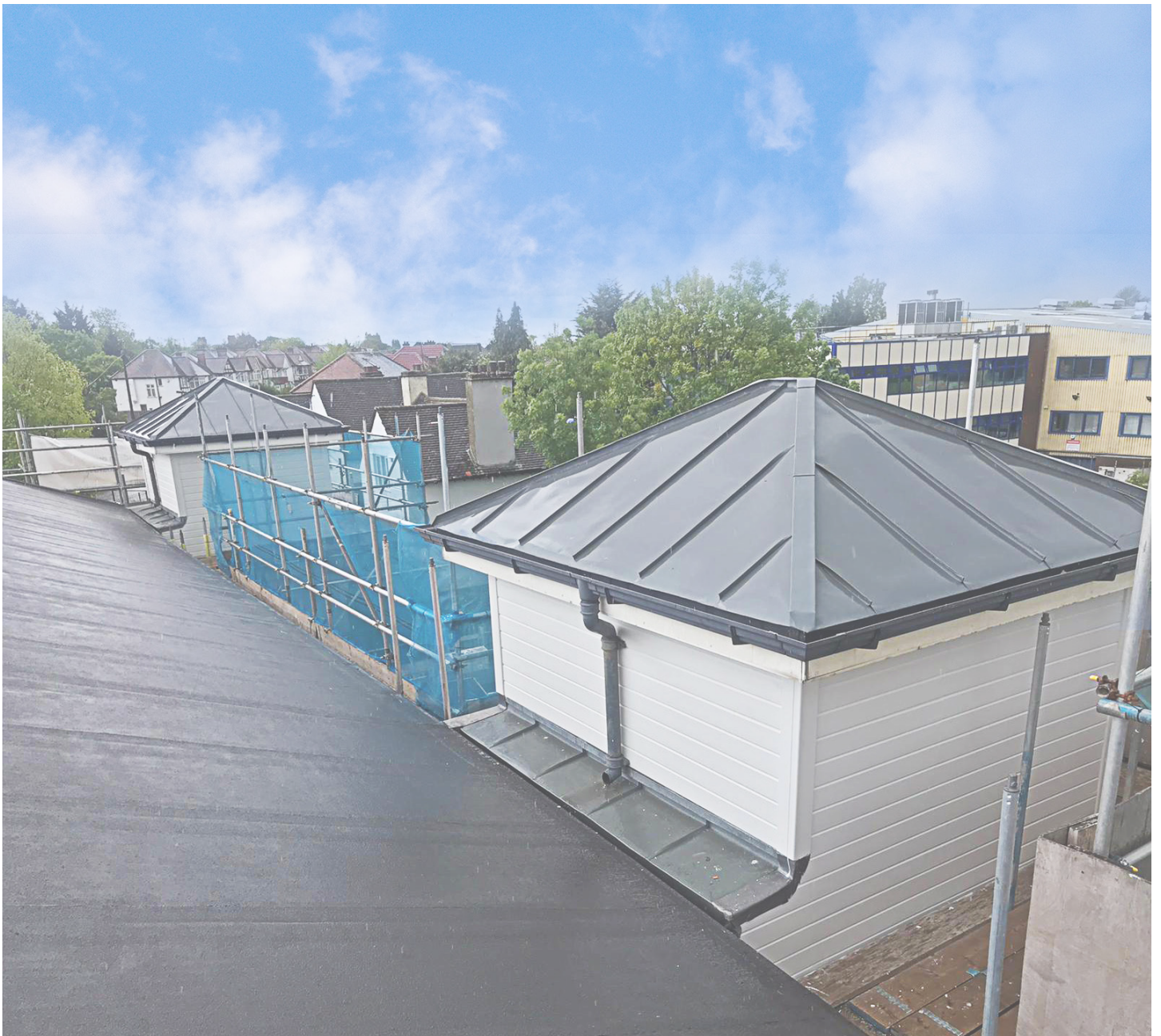
Roofing Details felt and standing seam
